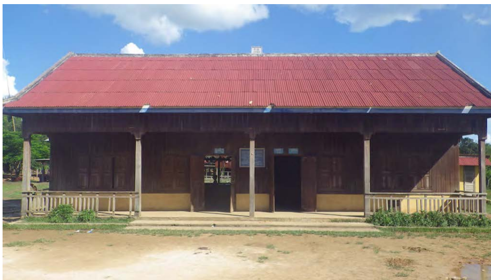
Figure 15. The Veal Denh School building in Anlong Chrey commune
